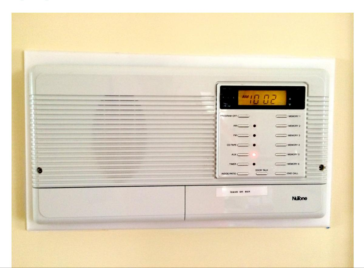
**Equipment:** intercom connected to a networked computer (now a Raspberry Pi running text-tospeech)
